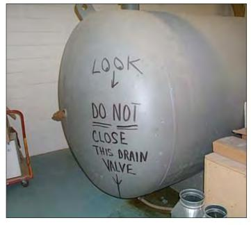
Figure 1: Manual valves left open waste huge amounts of energy.
