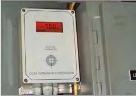
Figure 2: Dew point on this dryer was always a rock solid -70°C.
